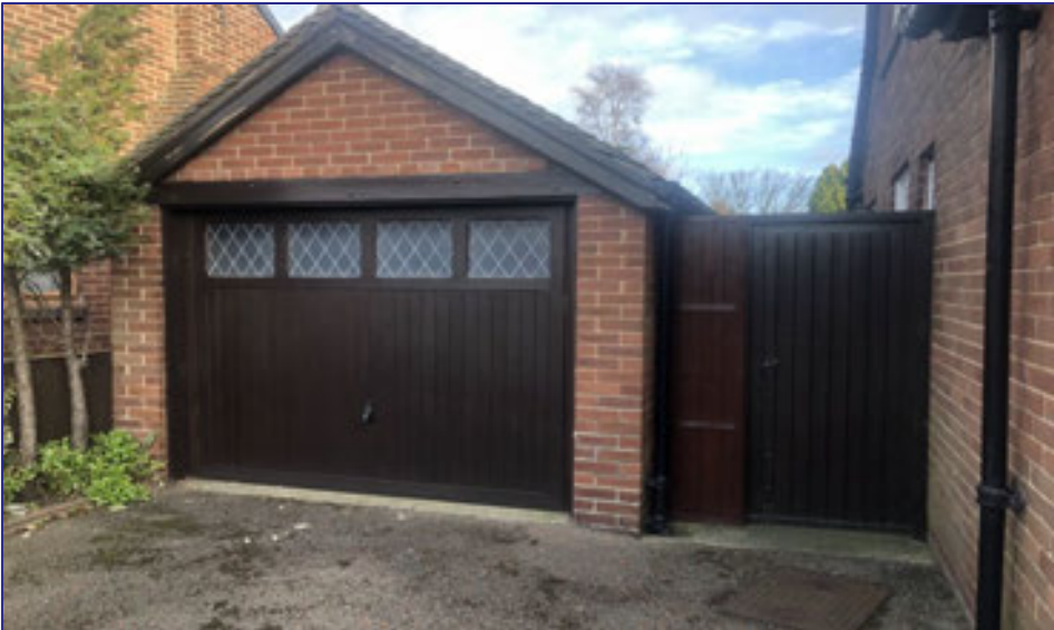
Photographic Plate 5 – Garage at top of drive, side of dwelling.
